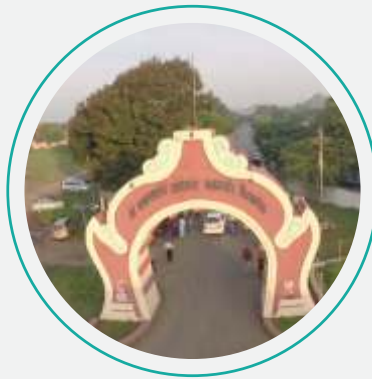
Aerial View of Main Entrance
