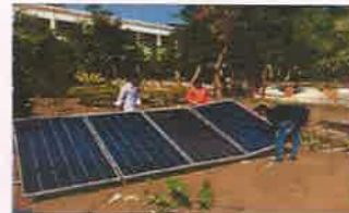
Field Installations for Training
