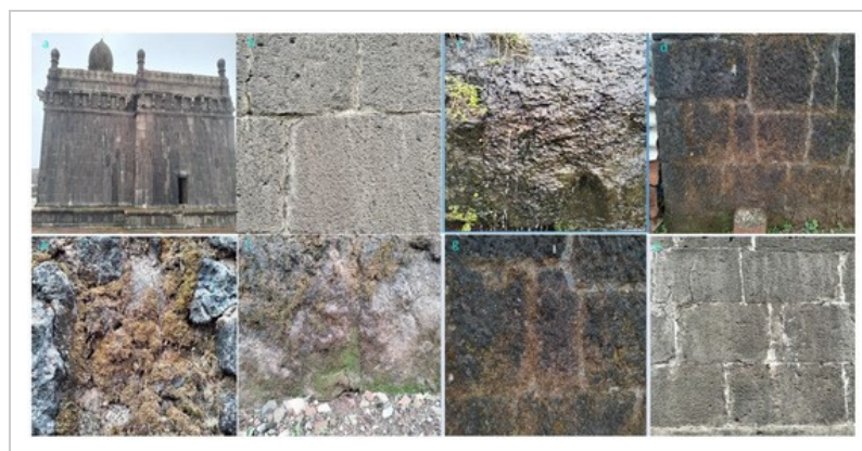
Figure 2. (a–h) showing stages of Ca-oxalate patina and their formation on basaltic stone surfaces, Raigad Fort.
